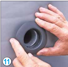
11 Put on the collars and push them onto the sockets
