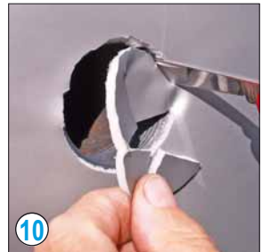
10 Carefully cut out the holes
