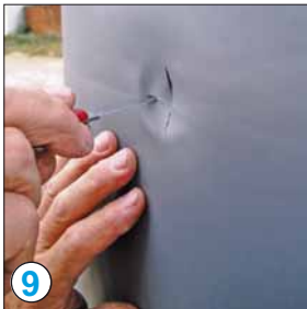
9 Feel for the sockets that are still underneath the PVC jacket
