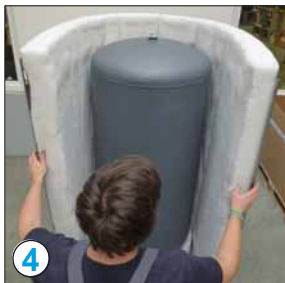
4 Tightly enclose the tank with the insulation
