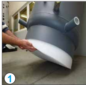
1 Tilt buffer tank and place bottom insulation underneath the tank
