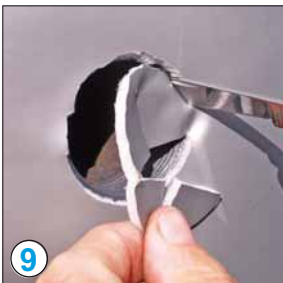
Carefully cut out holes
