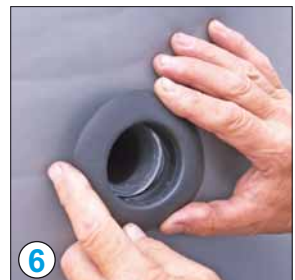
Put on the collars and push them onto the sockets
