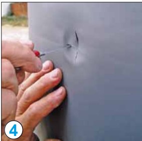
Feel for the sockets that are still underneath the PVC jacket
