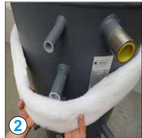
2 Pull the insulation ring for the tank's pedestal from top ...
