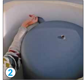
Adjust sockets to insulation
