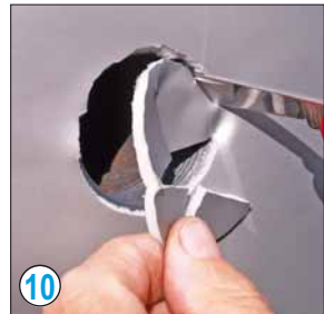
10 Carefully cut out the holes
