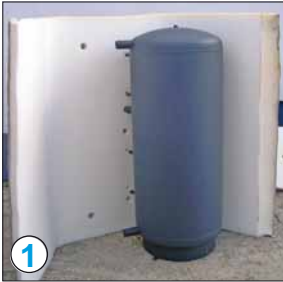
Only mount insulation when pre-heated. Pre-heat the insulation for at least 24 hrs to at least 22 °C.
