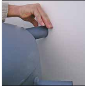
Only mount insulation when pre-heated. Pre-heat the insulation for at least 24 hrs to at least 22 °C.
